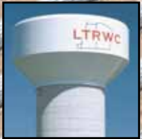
Potable Water Tanks
